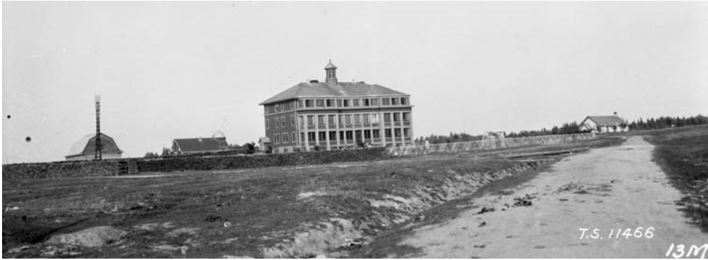
Figure A.35. Distant view of Norway House Indian Residential School, Norway House, Manitoba, 1927 (“C.S. Macdonald, Canada Department of Mines and Technical Surveys,” file PA-020236, LAC).
