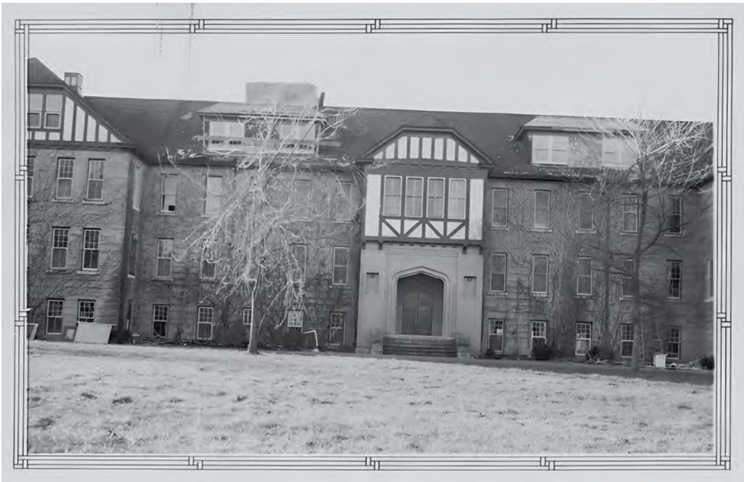
Figure 3.12. Coqualeetza Indian Hospital, front elevation showing new dormers, Sardis, British Columbia, January 11, 1941 (file e011080334, Department of Indian and Northern Affairs, LAC).
