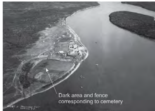
Figure 1.13. Annotated aerial photograph taken on July 12, 1930, of Fort Providence showing the location of the cemetery. Note the dark area (disturbed surface) on the field where the cemetery was located (Albert Lafferty, Chris Hugenholtz, Brian Moorman, and Thomas Andrews, "Integrating Geomatics, Geophysics, and Local Knowledge to Relocate the Original Fort Providence Cemetery, Northwest Territories," Arctic 74, no. 3 (2021): 407; created with photo no. A2567-11, National Air Photo Library).
