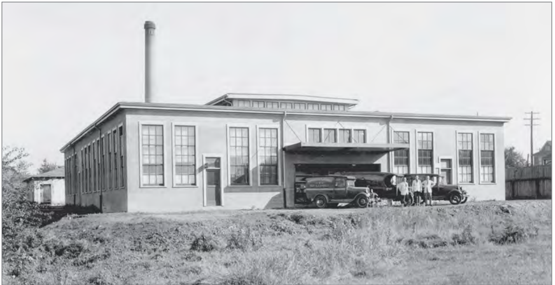
Figure 2.12. Blanchisserie du monastère et pressing, Vancouver (de « Sheet Metal Work: Monastery Laundry and Dry Cleaners at 562 West 14th Avenue », 1931, CVA 99-4054, Vancouver City Archives, https://searcharchives.vancouver.ca/sheet-metal-work-monastery-laundry-and-dry-cleaners-at-562-west-14th-avenue ).
